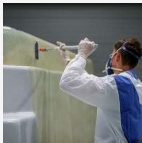
3. Application of an anti-corrosion fibreglass cloth
