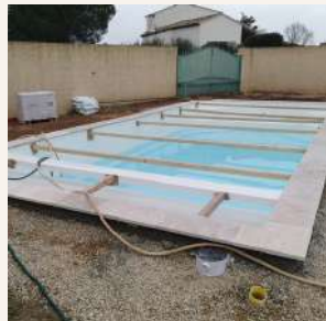
6. Laying coping stones* and putting in water
